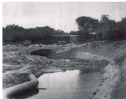
Construction of the Bronx River Parkway in the 1920s altered the path of the Bronx River.
