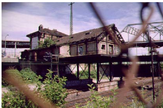
View of the Cass Gilbert station from the Concrete Plant Park.
