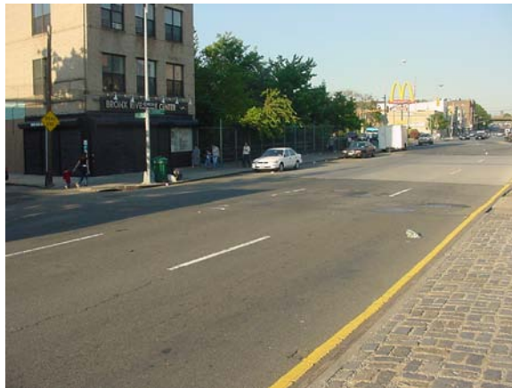
New curb "bulb outs" in front of the Bronx River Art Center will provide a safer crossing of E. Tremont Avenue, green the street, and promote stormwater capture.
