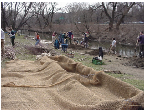
Volunteers lay bio-fabric along the Bronx River's shores in Shoe-lace Park to prevent bank erosion.
