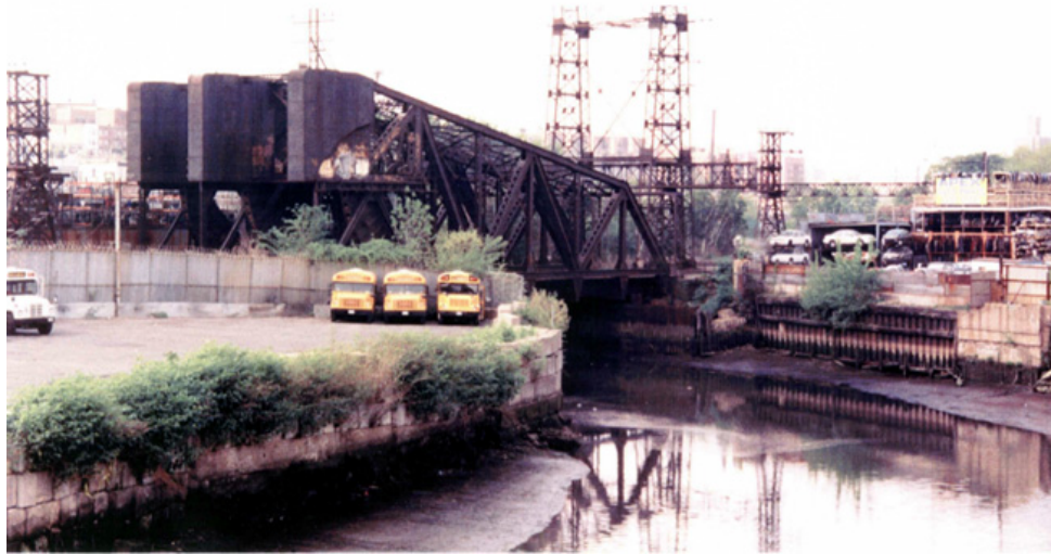
View of PDJ Simone and Apex properties from Westchester Avenue, looking north—before greenway construction (photo from NYSDOT)
