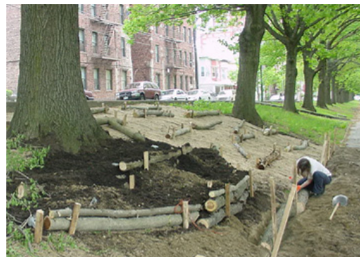
An upland erosion-control project in Shoe-lace Park stabilizes the slope down to the river.
