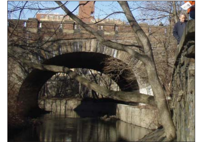
The historic bridge at Gun Hill Road
