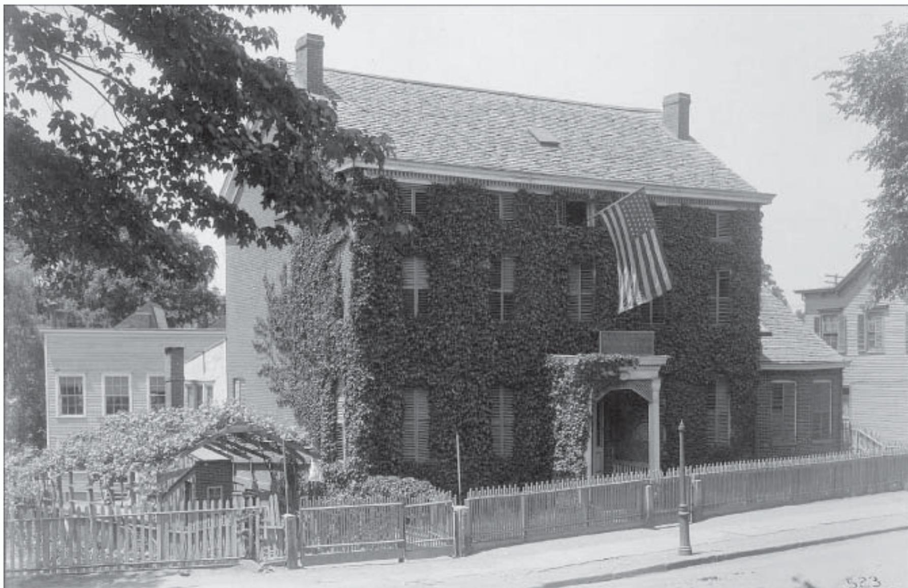
Williamsbridge Tapestry Works building (formerly Hotel Gorbets), 1913
