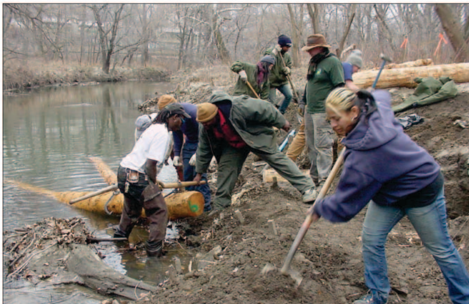
Construction of the Fort Knox Boat Launch, 2006
