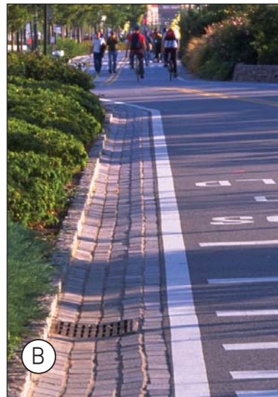
B Armorized swale adjacent to pavement
