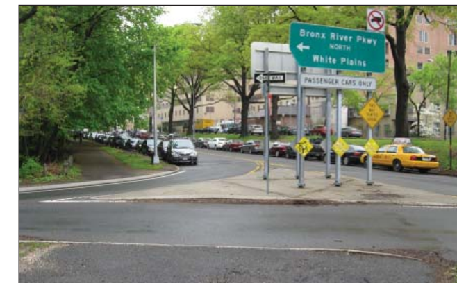
B. Existing conditions at on-ramp crossing
