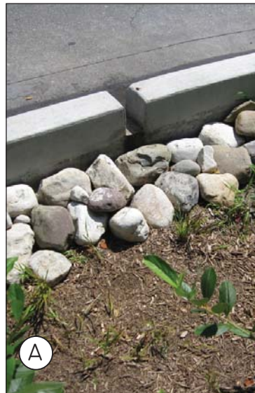
A Slotted curb and flow spreader
