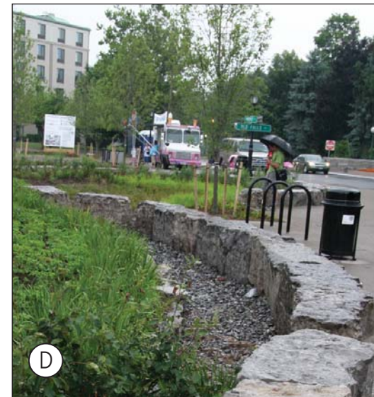
D Bioretention adjacent to paved area
