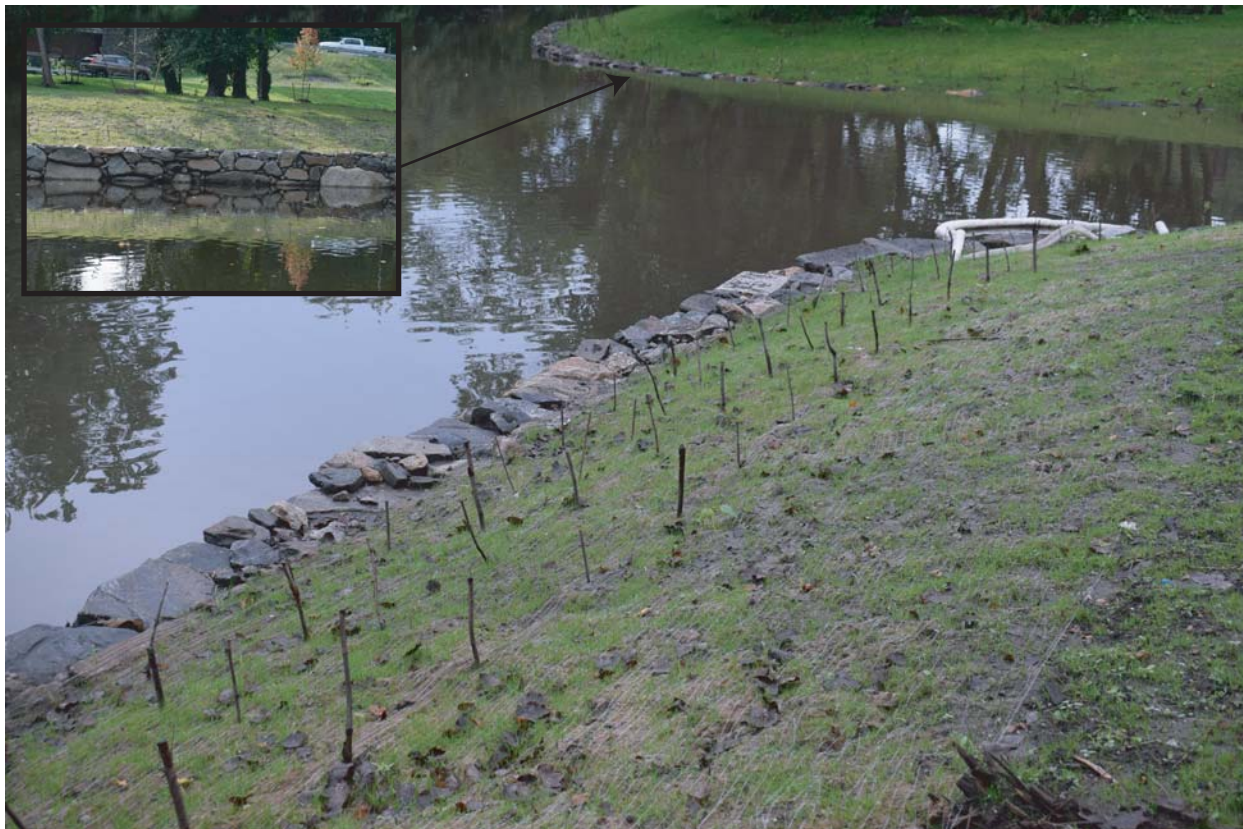
Figure 27. On Grassy Sprain Brook, a) armoring and straightening may be increasing sediment transport and bank instability downstream that led to b) construction of a bioengineering project at the confluence with the Bronx River.
