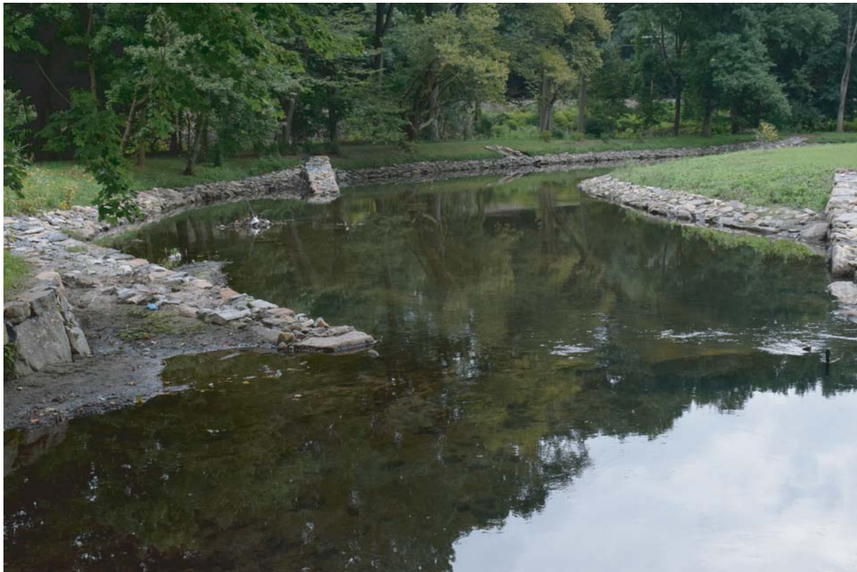
Figure 22. a) Deposition upstream and b) bank armor downstream (to arrest previous erosion) of the check dam at Harney Road.
