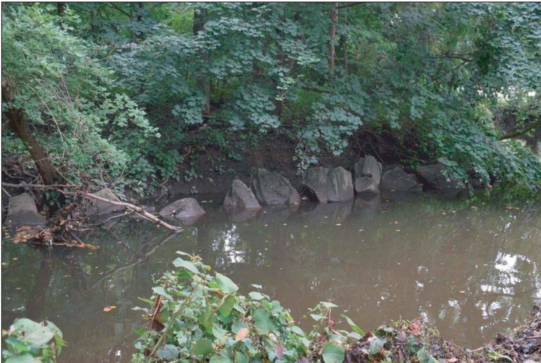
Figure 21. Erosion attacking a bank where the armor has failed on the Bronx River.
