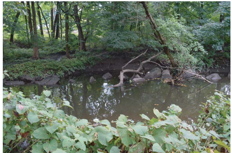
Failed bank armor has been outflanked along the remeandering channel (BR10I)
