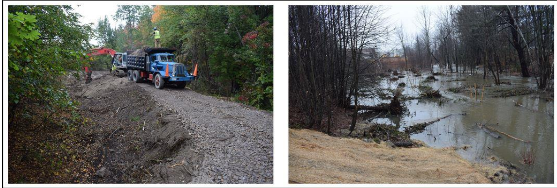
Figure 3. Berm removal (left) on Long Creek floodplain in October 2019 in South Portland, ME resulted in flow on the floodplain for the first time in more than 40 years (right) less than two months later during December 2019 rainstorm.
