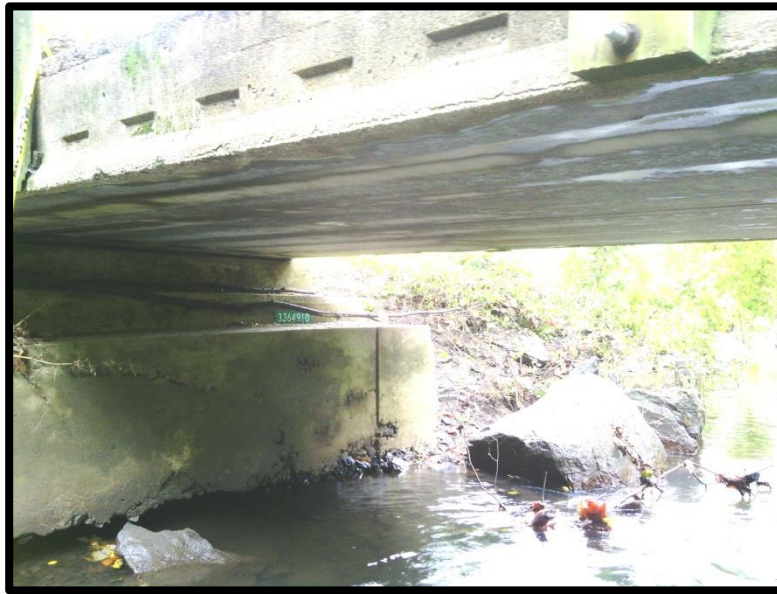
Figure A2-1: Photo of erosion removing protective material at a bridge on the Bronx River (BIN 3364910), leading to cracking of abutment's concrete.
