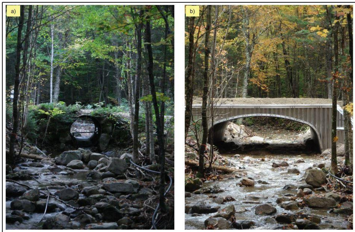
Figure 7. Paired photographs of a stream crossing on Long Mountain Brook in Coös County, NH a) before and b) after resizing the span in September 2008 to accommodate the channel's bankfull dimensions.
