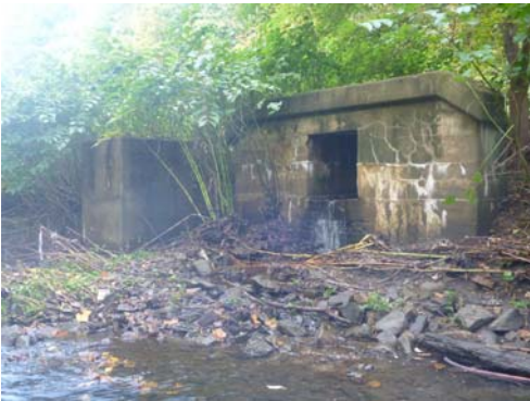
Stormwater outfall structures (BR_13A)
