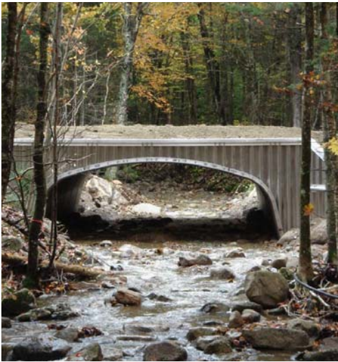
After: Properly sized stream crossing (22 ft span) (Coos County, NH)
