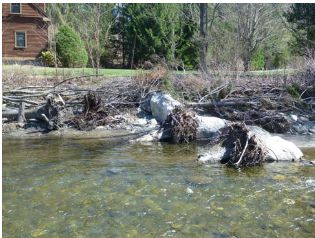
Boulder deflectors with log supports (South River, Conway, MA)
