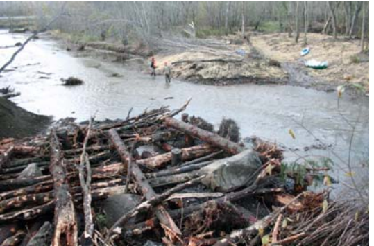
Log jams diverting flow into an abandoned meander along a straightened channel (Mohawk River, Colebrook, NH)
