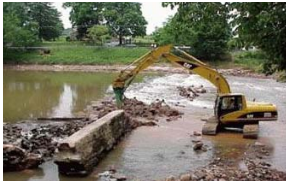
Removal of a concrete check dam ( http://ctfishing.blogspot.com/2005/06/old-dam-removal-before-after-pictures.html )
