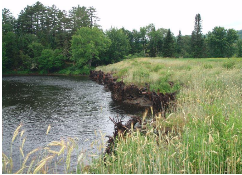
Figure 10. A series of marginal log jams protecting an eroding bank on the Connecticut River in Columbia, NH one year after construction.
