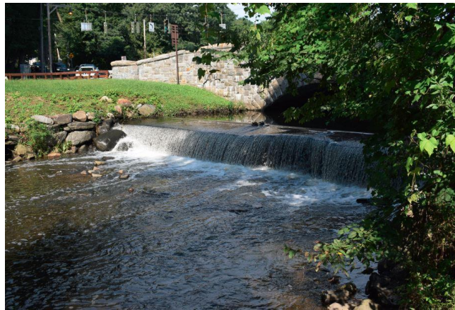
Figure 4. Check dam downstream of Harney Road fully blocks the channel. Note bank armor extending downstream.
