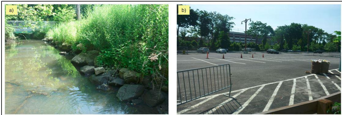
Figure 22. The Fisher Lane/North White Plains Station restoration reach showing a) the armor protecting the bank of artificial fill downstream of Fisher Lane (upstream view) and b) the parking lot built on that fill where the Bronx River used to flow prior to filling.
