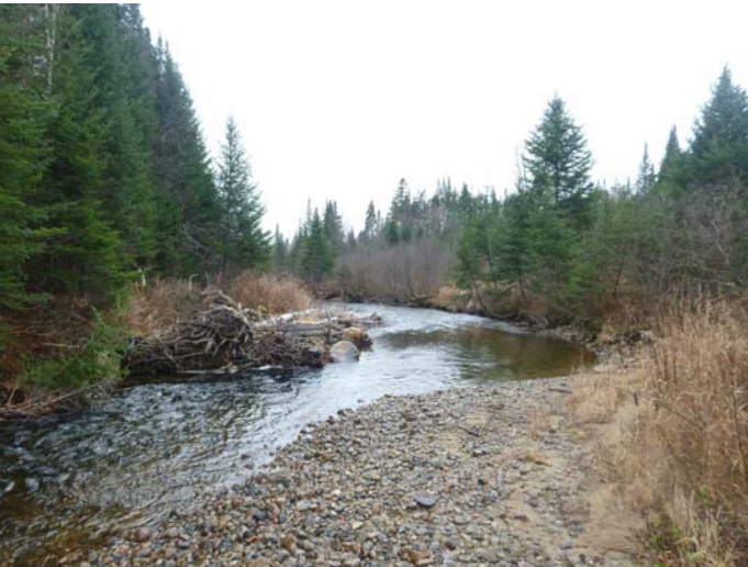
Constructing log jams to encourage meander growth (Nash Stream, Stark, NH)
