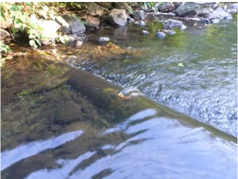
Sewer line crossing channel (BR_10A)
