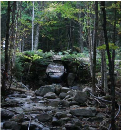
Before: Undersized stream crossing (6ft diameter) (Coos County, NH)
