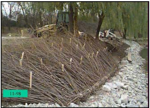
Brush mattress sample photo from National Engineering Handbook, Streambank Soil Bioengineering Technical Supplement 14I
