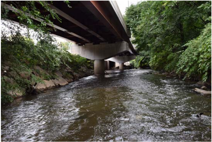
Viaduct carrying portion of Parkway over channel in Mount Vernon (BR_02A). Similar viaducts could elevate parkway above floodplain.
