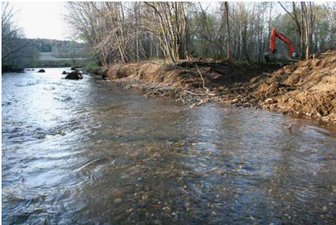
Diverting flow into an abandoned meander (Mohawk River, Colebrook, NH)
