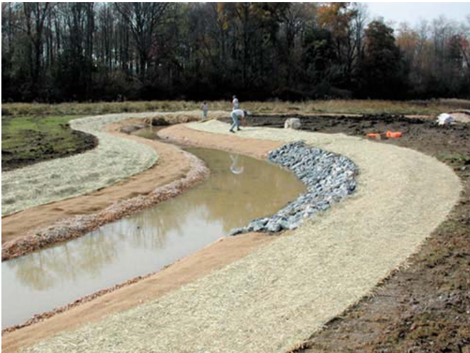
Excavating meanders utilizing natural channel design principles ( http://www.landandwater.com/features/vol46no2/vol46no2_1.html )
