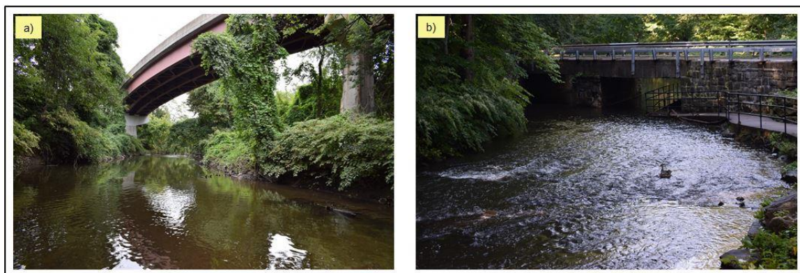
Figure 5. Some bridges a) fully span the bankfull channel of the Bronx River (Grassy Sprain Parkway) while b) others have spans narrower than the channel’s bankfull width (Northbound lanes of Parkway in Garth Woods).
